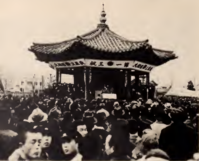
Tower in Pagoda Park in Seoul, which was the scene of mass demonstration in 1919 uprising
